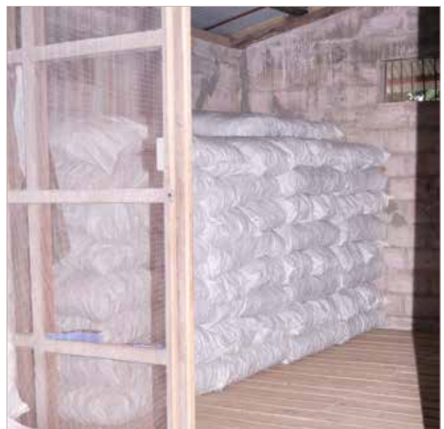
Bags in storage at an exporter's facility, showing mesh walls and grill windows for good ventilation
