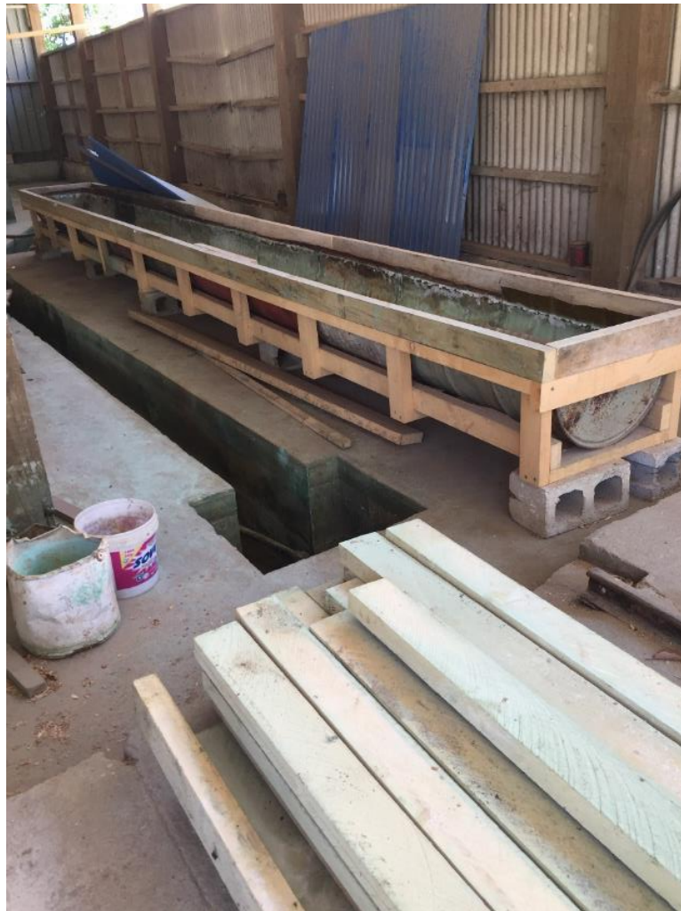
Figure 3-1 Basic 'dip' for preservative treatment of Vanuatu Whitewood on Efate
